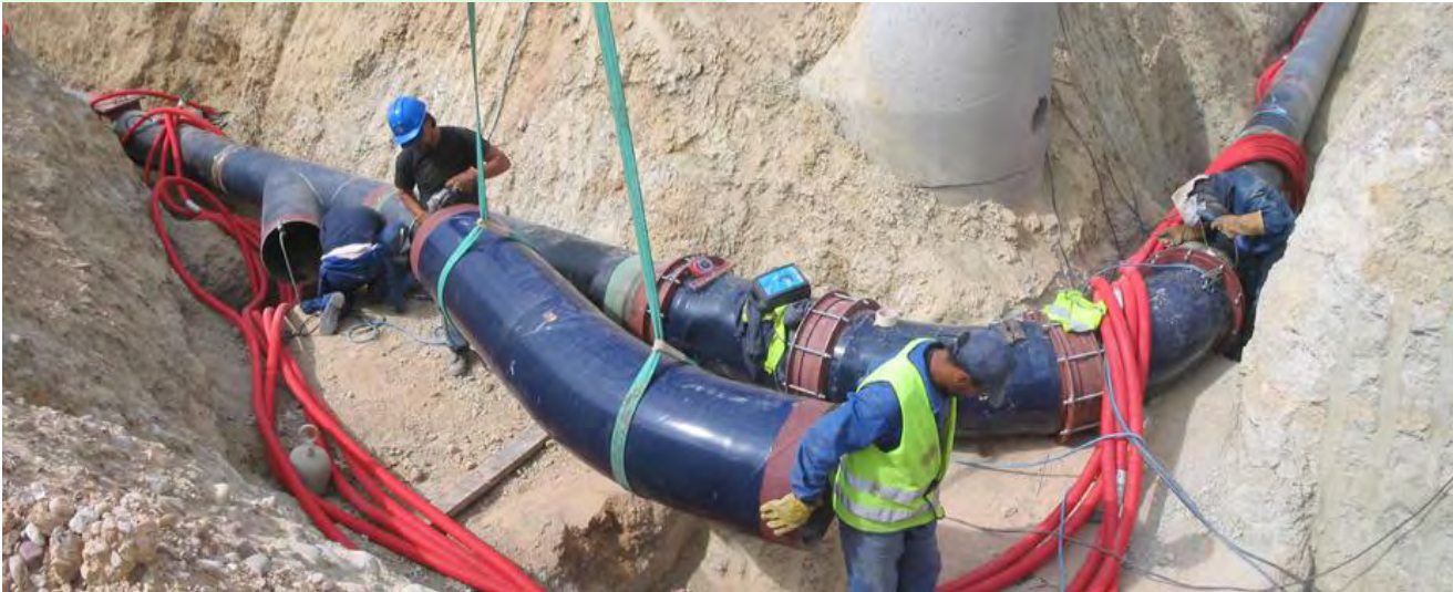
UNIÓN OF BRANCH R.II/3 WITH COLLECTOR II
