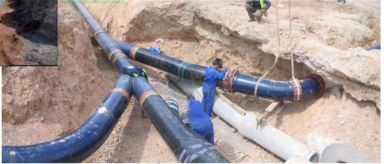
UNIÓN OF BRANCH R.II/3 WITH COLLECTOR II
